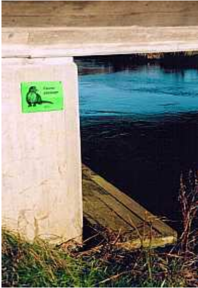
Pontoon underpass in Denmark pontoons (fot. Olimpia Pabian)
