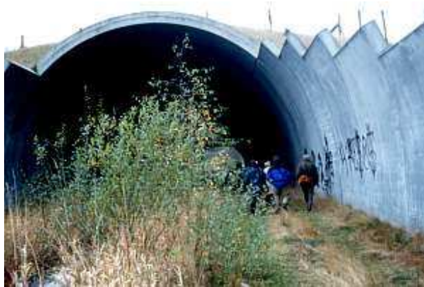
Oversized culvert as fauna underpass through a dam. (fot. Piotr Galicki)
