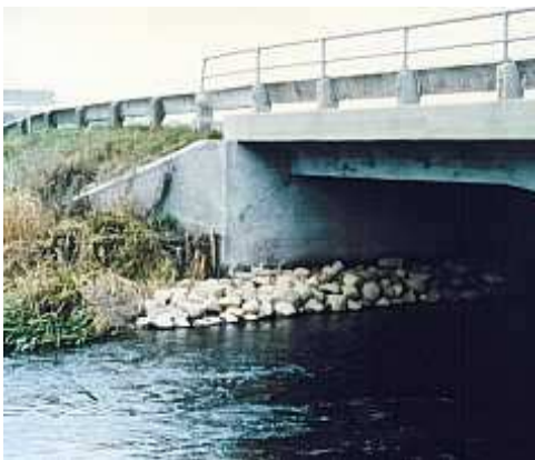
Fauna underpass constructed of boulders (fot. Aksel Bo Madsen)
