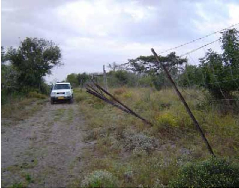
**Fig. 8. The fence, erected in 1998, has been broken by elephant because the solar panels, energizers and batteries were stolen.**
