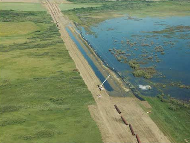
PHOTO 5-7: Typical Open Trench Construction across a Wetland
