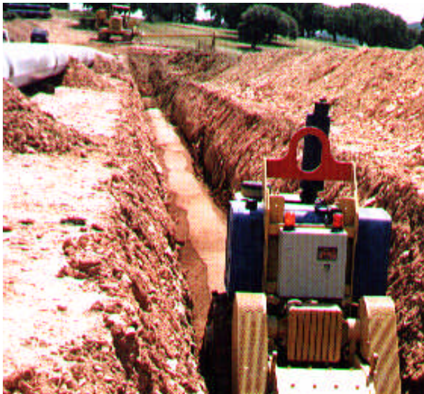
PHOTO 5-2: Bedding Machine used to compact the spoil
