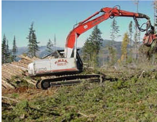
PHOTO 5-1: Typical Clearing Activities
