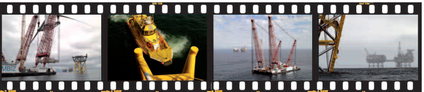
1-2 JULY 2007 Installation of Turbine B onto existing jacket installed in July 2006.
