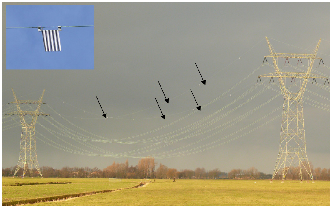
Figure 12. High-tension (150 kV) power line in the Netherlands with bird flappers (inset) (see arrows) placed at regular intervals in both ground wires as bird flight diverters, see also Box 1 (Photo: Bureau Waardenburg).
