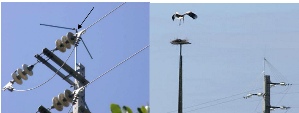
Figure 5. Distribution pole with symmetric chevron (arrow) on top as bird exclusion device (Photo: EDP-Distribution, Portugal) and dedicated nesting pole for White Stork next to distribution pole with bird exclusion device (Photo: Carlos Tiago).
